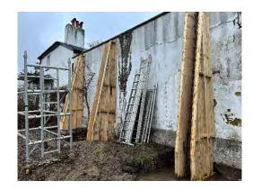
Work is underway to make safe a section of wall by building buttresses on the inside. The Garden remained closed whilst this work was undertaken.
